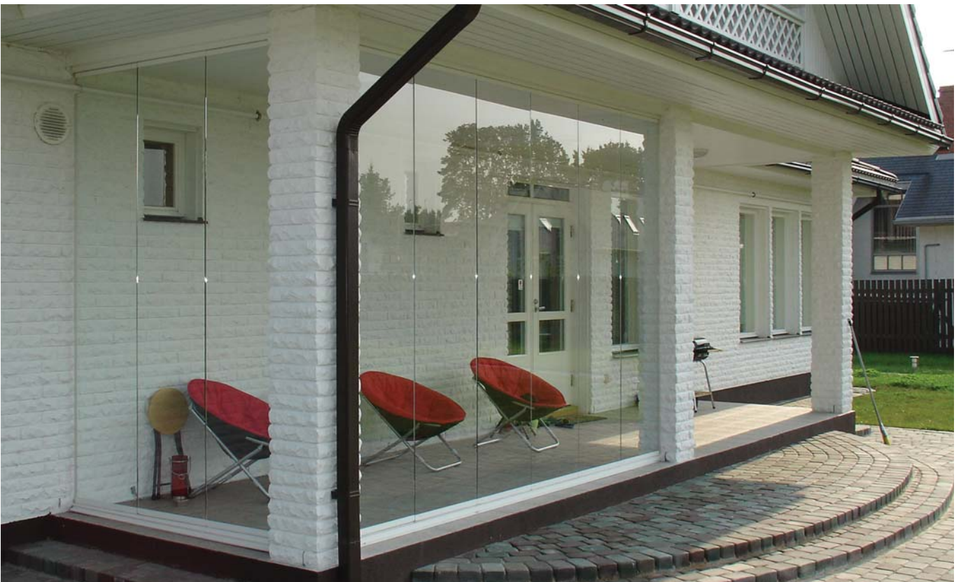
lestiklota āra terase Glazed exterior terrace
